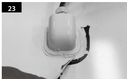
Remove friction tape .
