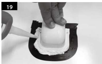
Apply silicone around the cable holder.
